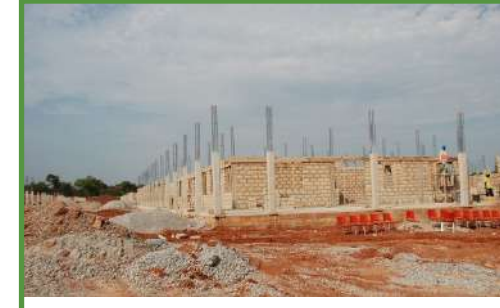
Hospital Emergency Block
