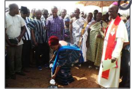
2019 Leyaata Hospital Groundbreaking
