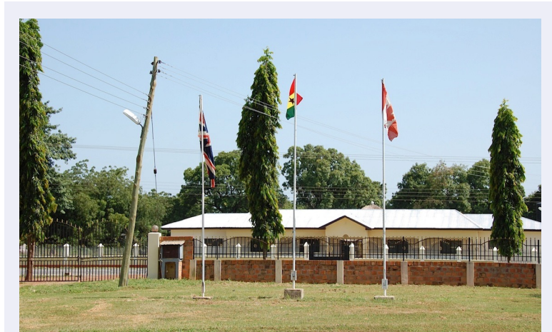
Team dorm at the NEA Project Site in Carpenter
